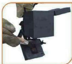
Step8.Clean the mold and proceed to the next solder joint operation
