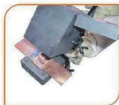
Step7.After 20 seconds, open the mold and clean the surface residue of the solder joint
