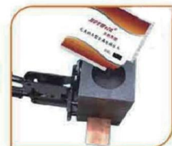
Step5.Place the welding powder into the mold. Place the kindling powder over the welding powder and leave a little over the mold mouth.
